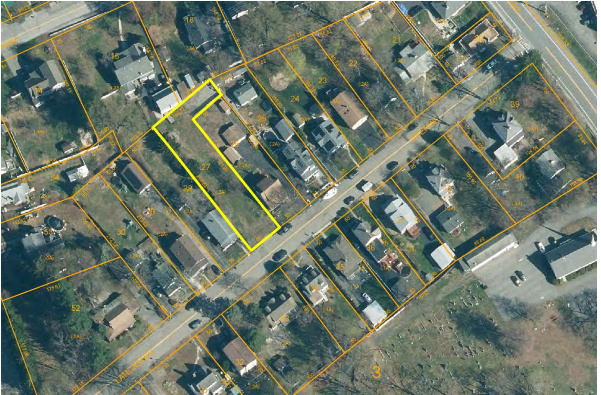
Aerial View, 0(17) Lancaster Avenue:
